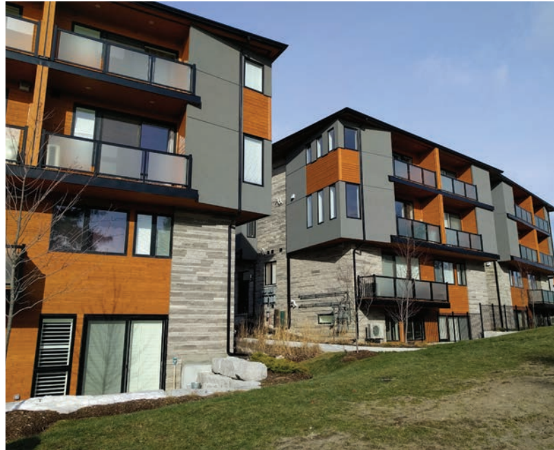
Existing townhouse development at Gordon St & Arkell Rd
