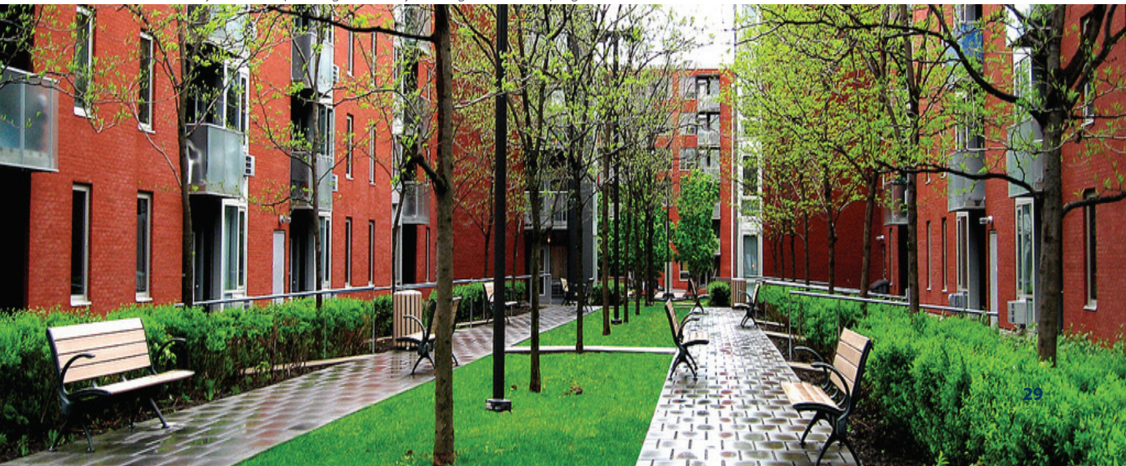
Common Amenity Area incorporating a walkway, seating and landscaping
