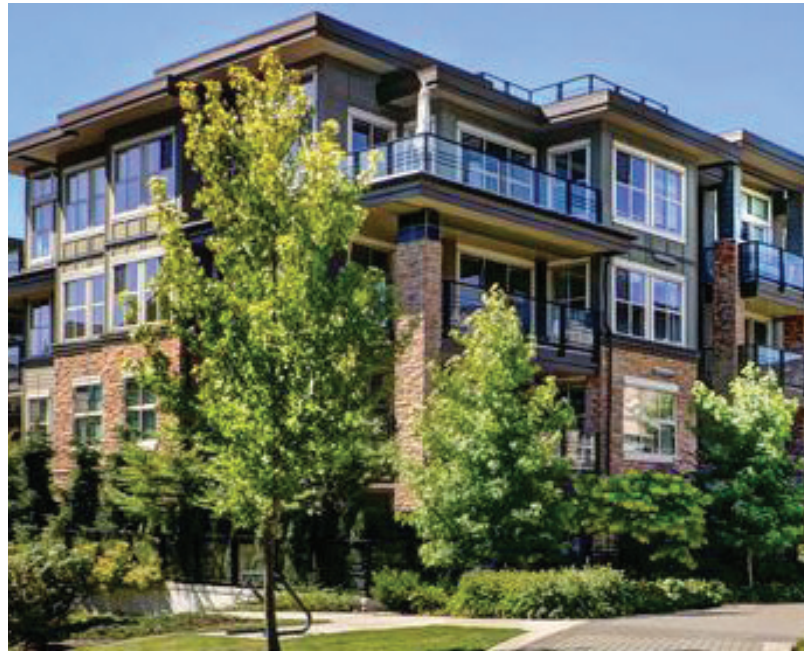
Townhouses development with articulated massing and landscaping
